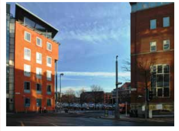
▲ Site as existing from Neville Street
